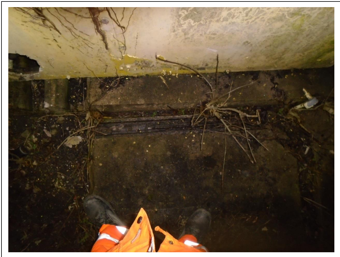
FIGURE 4: CONFIRMED ASBESTOS IN CEMENT TROUGHING IN SWITCH KIOSK - DESCRIPTION & RESULT OF ASSESSMENT (SAMPLE REF. 160000/050317/04)
