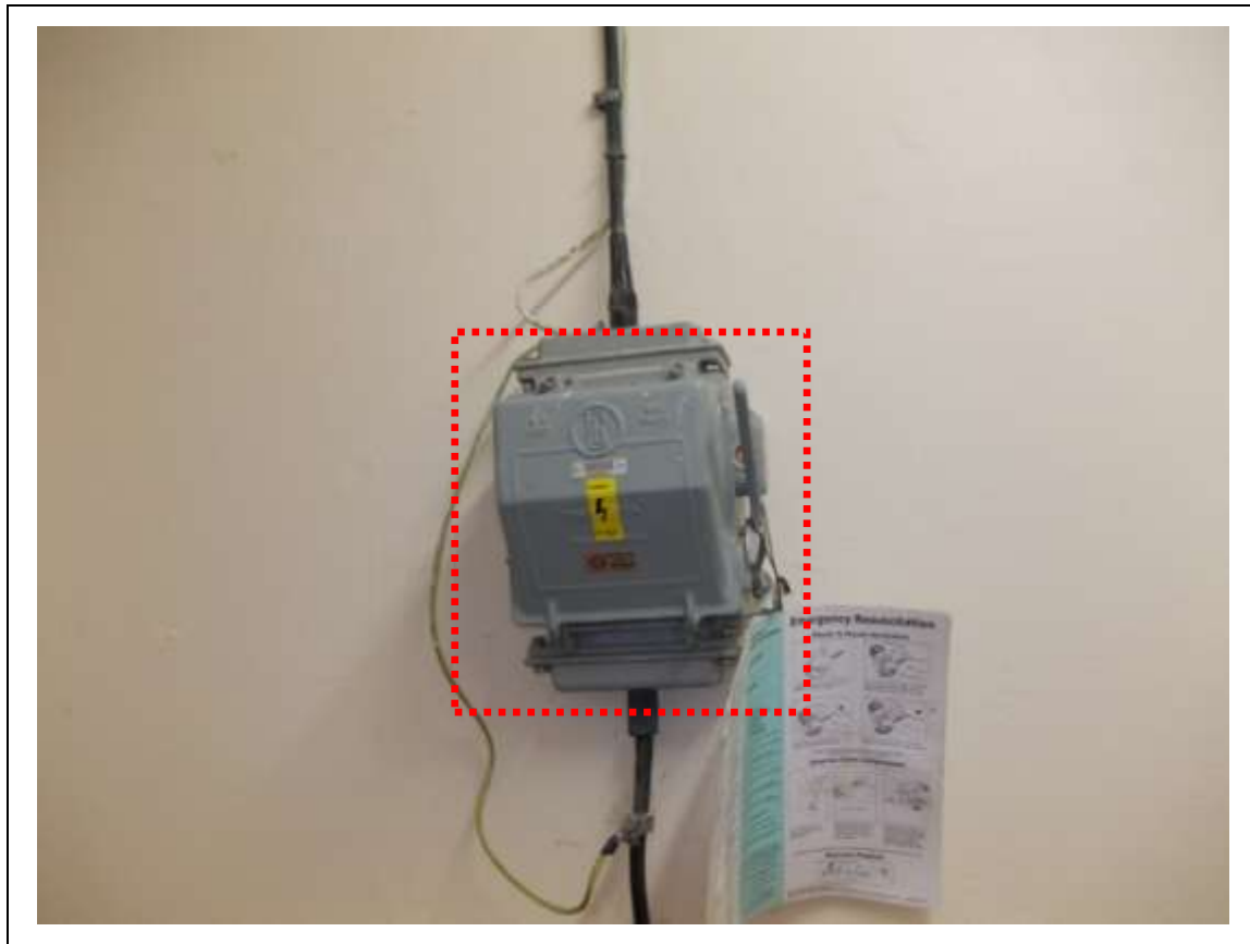
FIGURE 2: PRESUMED ASBESTOS IN MATERIALS WITHIN COMBINATION FUSE SWITCH BOX IN 0/081 - DESCRIPTION & RESULT OF ASSESSMENT (SAMPLE REF. P1 (2))
