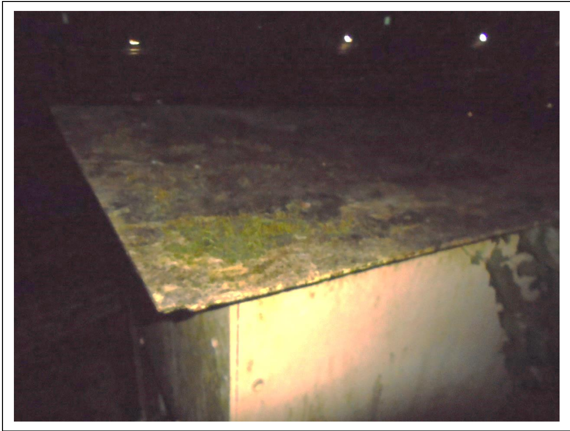
FIGURE 2: CONFIRMED ASBESTOS IN INSULATION BOARD PANELS IN SWITCH KIOSK - DESCRIPTION & RESULT OF ASSESSMENT (SAMPLE REF. 160000/050317/02)
