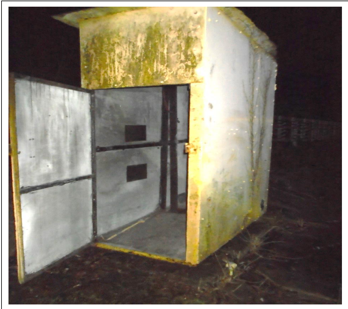
FIGURE 1: CONFIRMED ASBESTOS IN INSULATION BOARD PANELS IN SWITCH KIOSK - DESCRIPTION & RESULT OF ASSESSMENT (SAMPLE REF. 160000/050317/01)
