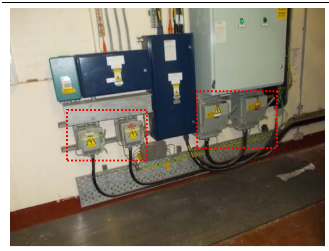
FIGURE 1: PRESUMED ASBESTOS IN MATERIALS WITHIN COMBINATION FUSE SWITCH BOXES IN UPS/ CONNECT, 0/662 - DESCRIPTION & RESULT OF ASSESSMENT (SAMPLE REF. P1 (1))
