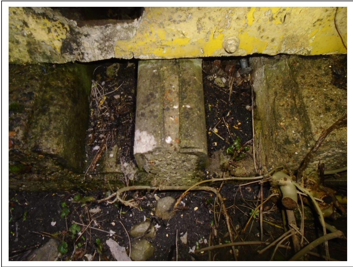
FIGURE 3: CONFIRMED ASBESTOS IN CEMENT TROUGHING IN SWITCH KIOSK - DESCRIPTION & RESULT OF ASSESSMENT (SAMPLE REF. 160000/050317/03)
