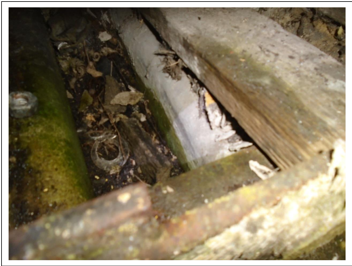
FIGURE 5: CONFIRMED ASBESTOS IN INSULATION BOARD DEBRIS IN SWITCH KIOSK - DESCRIPTION & RESULT OF ASSESSMENT (SAMPLE REF. 160000/050317/05)
